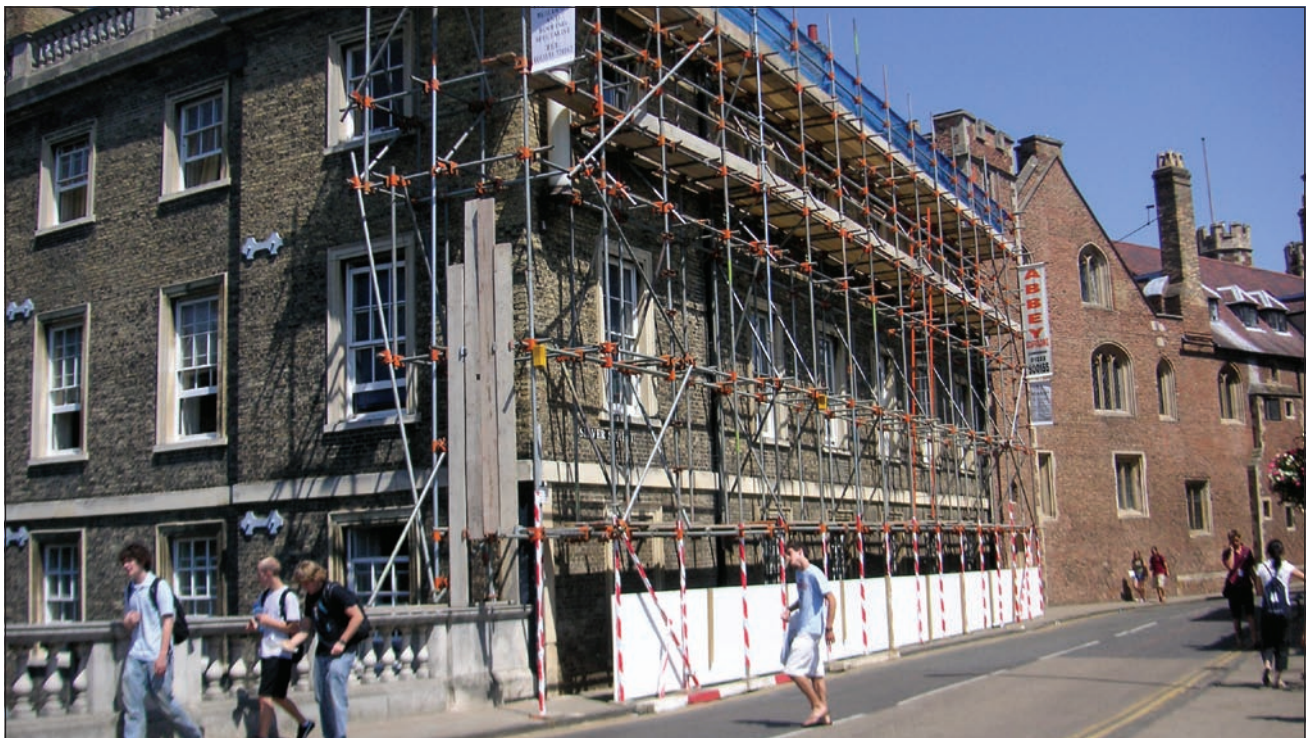
Repairs to the parapet of the Essex Building.
